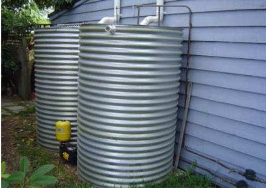
Figure 4: Picture of rainwater tanks
